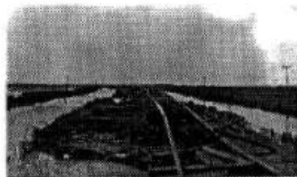
The flood of 1913 not only flooded homes, streets and crop land but the train rail bed also suffered heavy damage.
